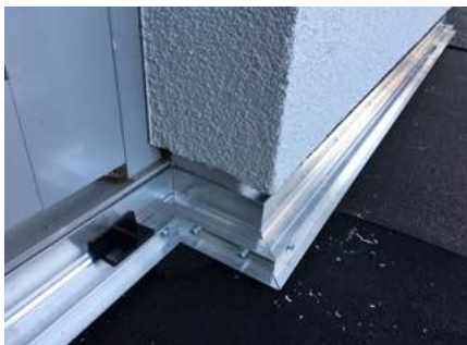
Bordering of a door niche in combination with external corner connectors and mitres cut to the edge profile
