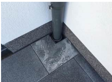
Recess for a downpipe with trimmed mitres and corner connectors
