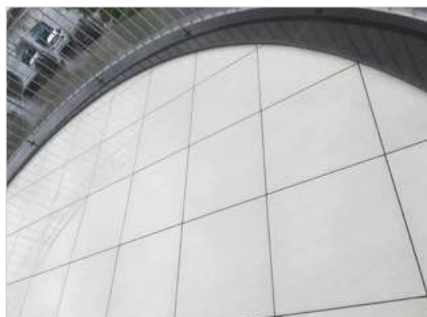
The TALUX slotted profile on a round surface with incised tile flooring
