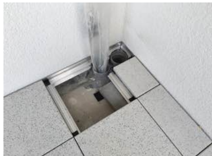
Cut-out for a downpipe with recessed TALUX edge profile
