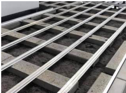
Height compensation with strip foundations, rubber pads and wedges
