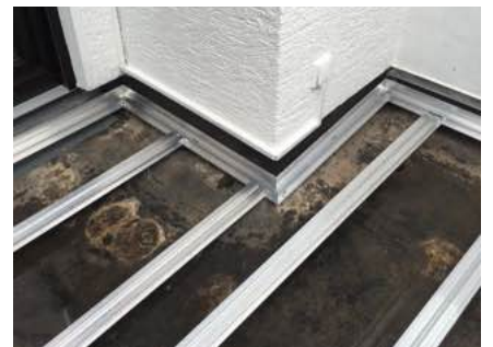
Circumferential bordering of an L-wall with the TALUX edge profile combined with external and interior corners
