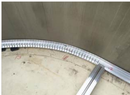
The TALUX slot profile to fit along a circular wall
