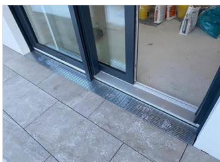
Drainage grating, resting on a TALUX system channel body
