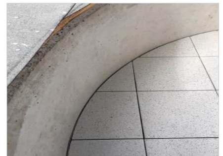
The TALUX slotted profile fitted along a circular wall with incised tile flooring
