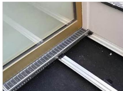
Drainage gutter, flush fitted into the TALUX system
