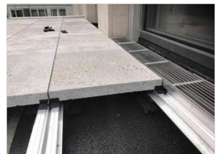
Drainage gutter, fitted to the side of the TALUX edge profile
