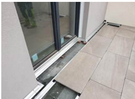
Bordering of a door niche with the TALUX edge profile combined with external and interior corners
