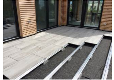
Height compensation with paving stones, rubber pads and wedges
